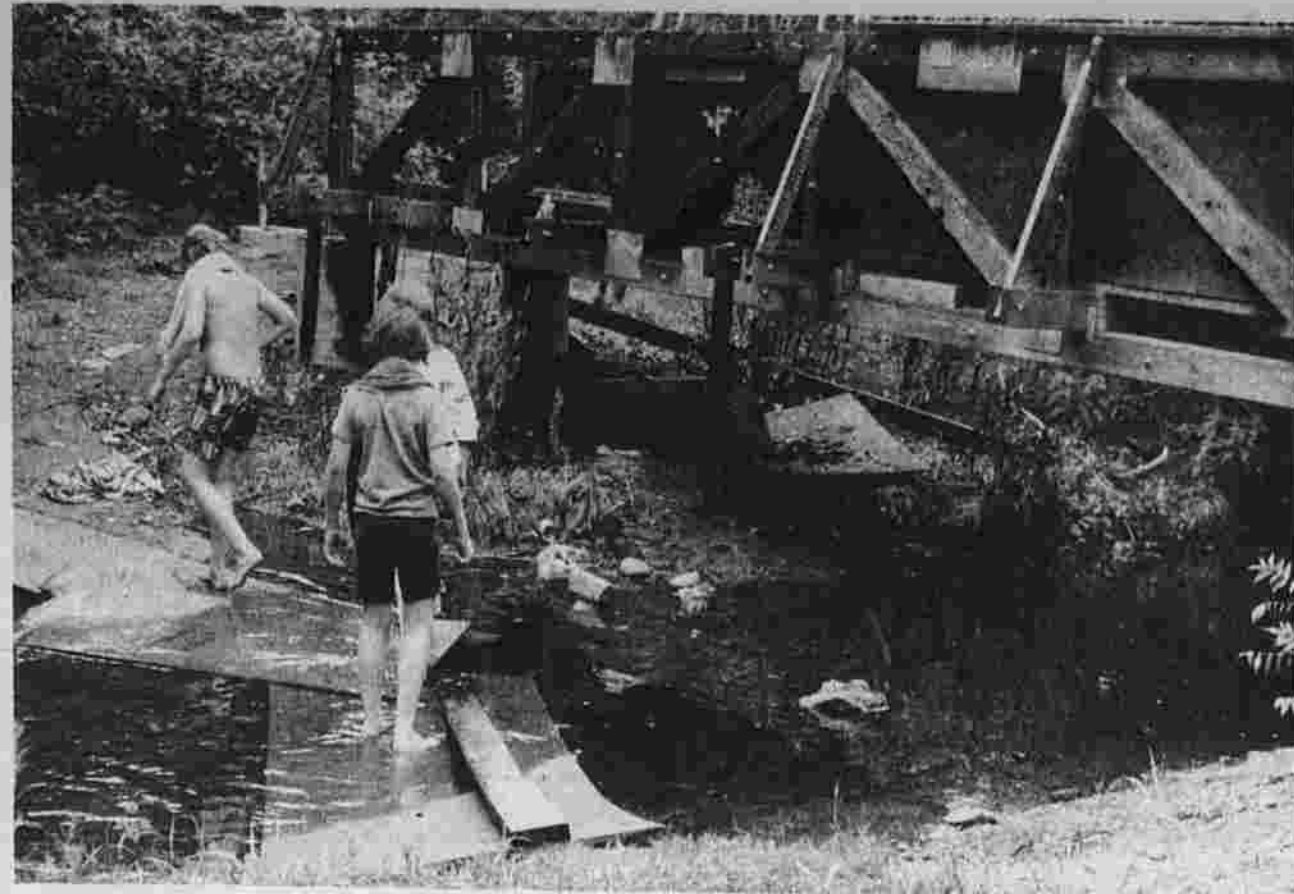
Bypassing Burned-Out Bridge
